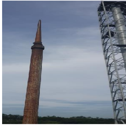
Gambar 2. Air termination
